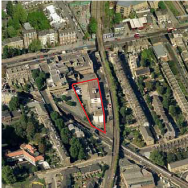
Aerial photo of site North ↑
